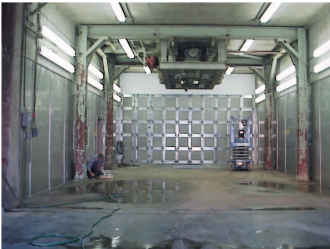
After/ Water Blast Room
